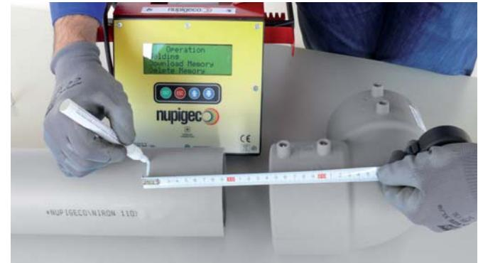
Insert the pipe or spigot ends into the fitting up to the marked insertion length. When necessary, position the aligners in order to maintain the position. Be sure to avoid any mechanical stress during the welding procedure and cooling time.
