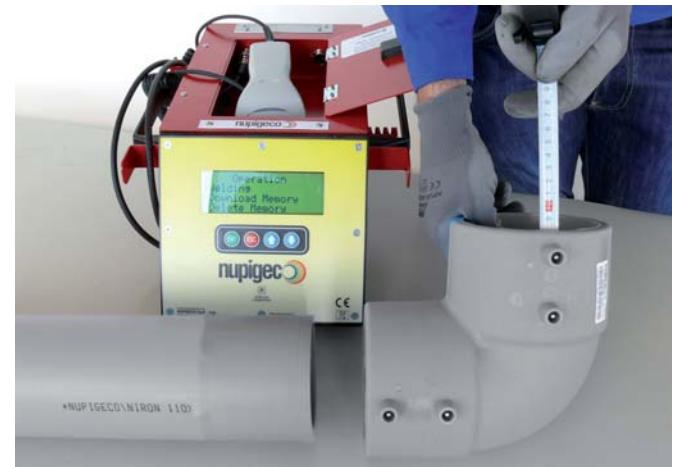
Mark the welding insertion depth on the pipe (equal to the length of the electrofusion fitting socket) with the appropriate marker.
