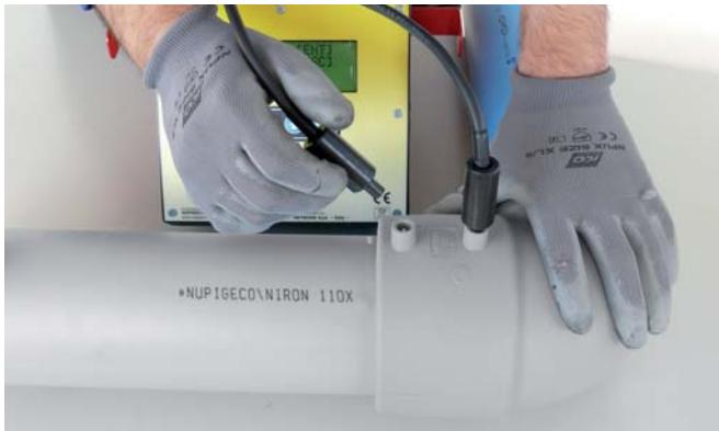
Prepare the pipe and fitting to be welded following the directions in the previous chapter. Make sure that the pipe and fitting to be welded are lined up without any possibility of movement (use a suitable aligner whenever it is possible or practical to do so).
