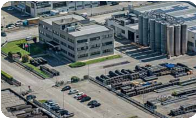
Production Facility - Castel Guelfo di Bologna (BO)
