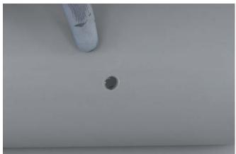
Once the heating time is over, insert the male cap inside the hole without rotating.
