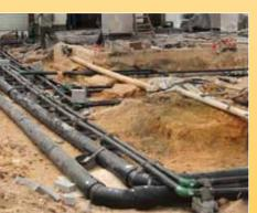
All the primary SMARTFLEX piping nsists of a composite-wall lined uct which, by combining the ent mechanical properties of HDPE with the low permeability and high resistance to hydro-carbons of a new ass of polymers, creates a level of ydro-carbon resistance unattainable by other fuel pipes on the marke
