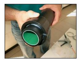
5. Fit the two metal clamps around the shells and tighten them evenly. Spread the excess adhesive around with a blade or spatula.
