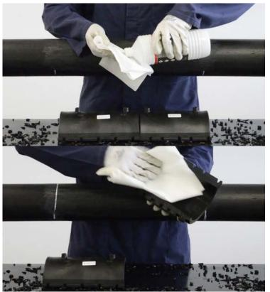
5 Mark on the scraped pipe a distance equal to the whole length of the assembled sleeves, so that the damage is well centered and surrounded. Take care not to contaminate the previously cleaned surfaces.
