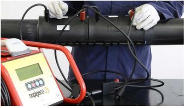
12 Perform welding: scan with the optical pen the barcode on EIVLRS I module and proceed with welding.
