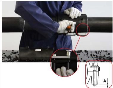
7 Place the terminal module EIVLRS **T** on the scraped pipe, adjacent to the previous one just installed: the lip at the end of the module must overlap the protruding edge of the previous one. Install the first underclamp across the two adjacent modules (follow the instruction on Step 6). Then install the second and third underclamps in the consecutive positions (follow the instruction on Step 6). The terminal module <u>EIVLRS **T**</u> must always be the final module installed.
