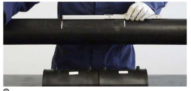
${f 2}$  Measure the total length of the sleeve modules and mark it on the pipe, beyond the damage. Maximum coverable area: 4": 4.17x12.36" (106x314 mm) - 2.36" from border 6": 4.50x12.36" (114x314 mm) - 2.36" from border max depth of damage: 25% of wall thickness of pipe.
