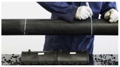
**(b)** <u>Install each single module separately on the pipe, starting</u> <u>from one end of the scraped area:</u> place the EIVLRS I module first on the pipe and align it to the marked line.
