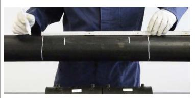
${\mathfrak B}$  Scrape the part of the pipe where the variable length repair sleeve will be welded, over and all along the damage to be repaired.
