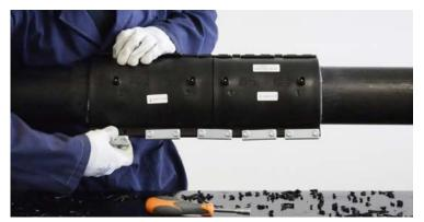
Before proceeding to Step 8 verify that all the underclamps are properly tightened (feel the screws sticking out of the bottom); eventually use a wrench to tighten the screws if necessary. Use caution when tightening screws. Power tools or excessive torque can result in damage.
