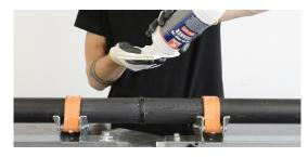
**5.** Clean also the inner surface of the fitting with the same isopropyl alcohol.
