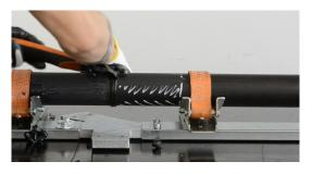
4. Clean the pipe surface with isopropyl alcohol (minimum concentration 91%).
