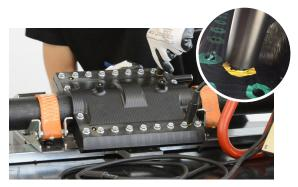
**11.** Connect the welding unit with the other two pins of the lateral zones. Scan the specific barcode of the <u>LATERAL ZONES</u> and start the welding.
