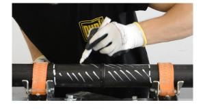
3. Scrape with a manual scraper the part of the pipe where the repair sleeve will be welded without removing the bead.
