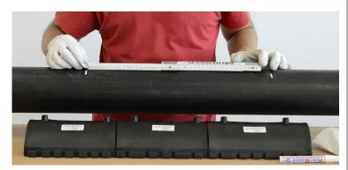
2 Measure the total length of the sleeve modules and mark it on the pipe, near the damage. Minimum distance required for the fitting to extend beyond the damaged area: 2,36" (60mm).
