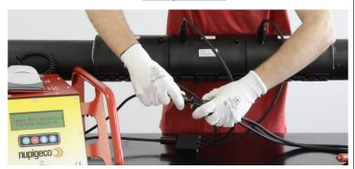
14 Connect each connector of the <u>red triple cable</u> to the second pin marked "B" of each module.
