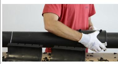
Place the first underclamp on the very end of the assembly: hook the square holes of the underclamp to the teeth on the side of the module; align the two screws to the corresponding holes, line up the metal spacer and use a wrench to tighten the two screws until they are in position A in the lower part (feel the screws sticking out of the bottom - see figure in the circles below). Repeat the operation with the second underclamp in the consecutive position.
