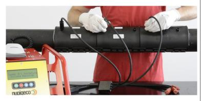
13 Connect the other cable of the electrofusion machine to the connector slot of the red triple cable.
