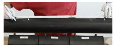
$rac{3}{2}$  Scrape the part of the pipe where the variable length repair sleeve will be welded, over and all along the damage to be repaired.
