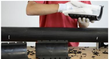
f 5 Mark on the scraped pipe a distance equal to the whole length of the assembled sleeves, so that the damage is well centered and surrounded. Take care not to contaminate the previously cleaned surfaces.
