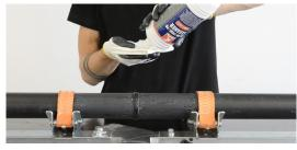
**5.** Clean also the inner surface of the fitting with the same isopropyl alcohol.
