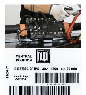
**15.** At the end of the second welding, mark again weld number and time on the body of the fitting and wait 30 minutes to allow the welded parts to cool down.
