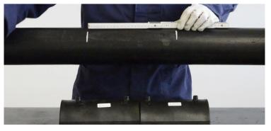
2 Measure the total length of the sleeve modules and mark it on the pipe, near the damage. <u>Minimum distance required for</u> the fitting to extend beyond the damaged area: 2,36" (60mm).
