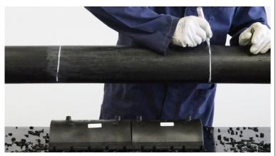
**(5)** Install each single module separately on the pipe, starting from one end of the scraped area: place the EIVLRS I module first on the pipe and align it to the marked line.
