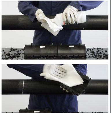
Mark on the scraped pipe a distance equal to the whole length of the assembled sleeves, so that the damage is well centered and surrounded. Take care not to contaminate the previously cleaned surfaces.
