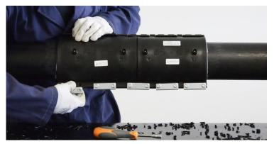
Before proceeding to Step 11 verify that all the underclamps are properly tightened (feel the screws sticking out of the bottom); eventually use a wrench to tighten the screws if necessary.
