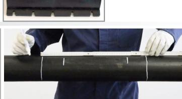
Scrape the part of the pipe where the variable length repair sleeve will be welded, over and all along the damage to be repaired.
