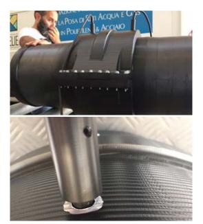
**15.** Wait 30 minutes to allow the welded parts to cool down. Restart with a new welding of the lateral zone repeating to the point 10 - 11 - 12.
