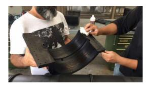
**6.** Install the two half shells on the pipe. Keeping the bead in the center.
