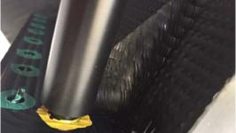
**16.** The alignment clamp can be removed 30 minutes after the last fusion is completed.
