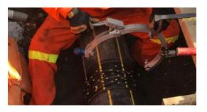
**4.** Clean the pipe surface with isopropyl alcohol (minimum concetration 91%).
