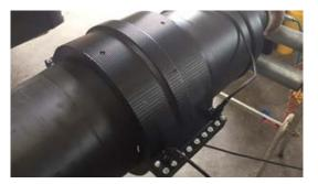
**13.** Using the jumper cable connect the two white pins of the central zones; connect the welding machine to the other 2 pins of the central zones.
