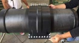
8. Using a screw driver tight the two shell together.
