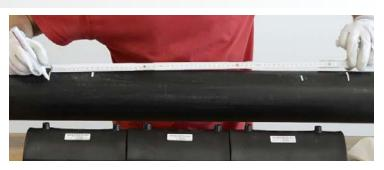
${rac{3}{3}}$  Scrape the part of the pipe where the variable length repair sleeve will be welded, over and all along the damage to be repaired.
