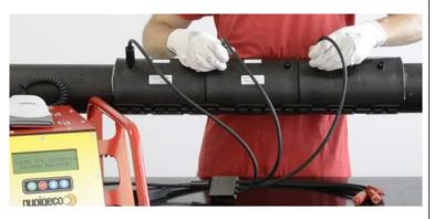
**13** Connect the other cable of the electrofusion machine to the connector slot of the <u>red triple cable</u>.
