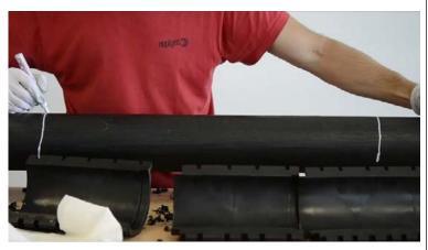
**(5** Install each single module separately on the pipe, starting from one end of the scraped area: place the EIVLRS I module on the pipe and align it to the marked line.
