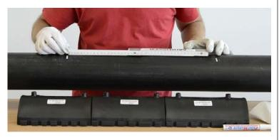
${f 2}$  Measure the total length of the sleeve modules and mark it on the pipe, near the damage. Minimum distance required for the fitting to extend beyond the damaged area: 2,36" (60mm).
