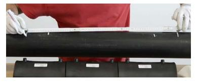
🕹 Scrape the part of the pipe where the variable length repair sleeve will be welded, over and all along the damage to be repaired.
