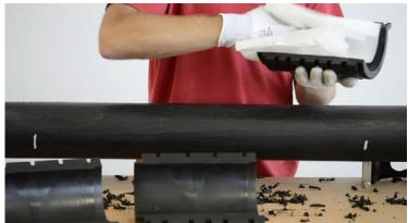
$oldsymbol{\mathfrak{G}}$  Mark on the scraped pipe a distance equal to the whole length of the assembled sleeves, so that the damage is well centered and surrounded. Take care not to contaminate the previously cleaned surfaces.
