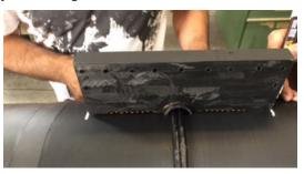
3. Scrape with a rotary scraper the part of the pipe where the repair sleeve will be welded without removing the bead.
