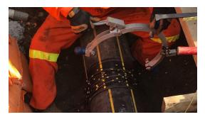
4. Clean the pipe surface with isopropyl alcohol (minimum concetration 91%).
