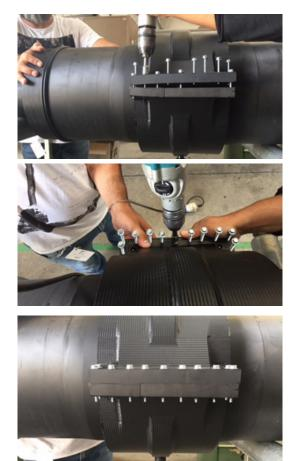
**9.** In any case before starting the fusion process, fit the alignment clamp and check if it is firmly secured on either side of the BFRS.
