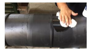
5. Clean the inner surface of the fitting with isopropyl alcohol (minimum concentration 91%).
