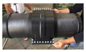
8. Using a screw driver tight the two shell together.
