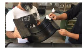
6. Install the two half shells on the pipe. Keeping the bead in the center.
