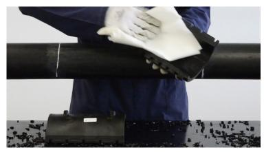
5 Mark on the scraped pipe a distance equal to the whole length of the assembled sleeves, so that the damage is well centered and surrounded. Take care not to contaminate the previously cleaned surfaces.
