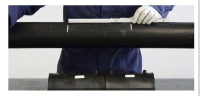
f Z Measure the total length of the sleeve modules and mark it on the pipe, near the damage. Minimum distance required for the fitting to extend beyond the damaged area: 2,36" (60mm).
