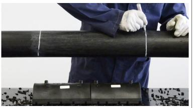
5 Install each single module separately on the pipe, starting from one end of the scraped area: place the EIVLRS I module first on the pipe and align it to the marked line.
