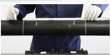
$rac{3}{3}$  Scrape the part of the pipe where the variable length repair sleeve will be welded, over and all along the damage to be repaired.
