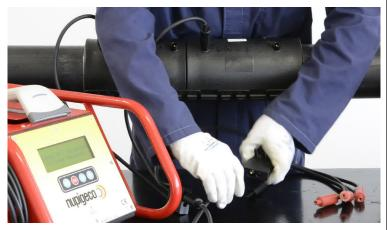
11 Connect 2 connectors of the <u>red triple cable</u> to the second pin marked "B" of each module. The third connector doesn't need to be used.
